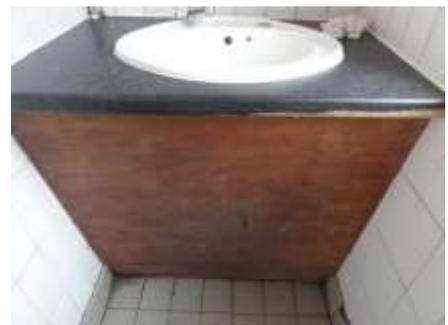
**Figure 6 Rotting and chipped sink unit**
